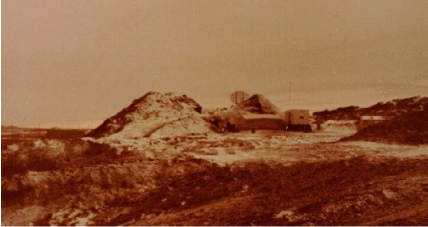
Radar TPS-43 Westinghouse, Río Grande (1982)
